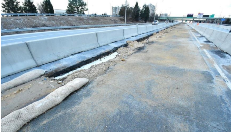
Work zone near Duke Street following the demolition of guardrail in anticipation of the addition of a new travel lane in the Express Lanes.
