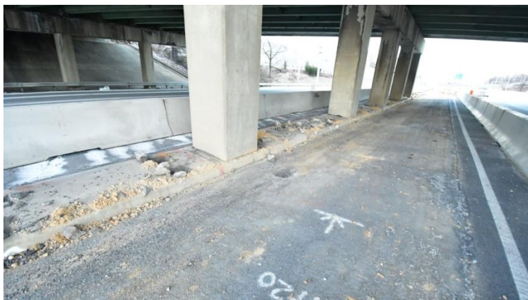
Bridge overpass maintenance work along the northbound I-395 general purpose lanes.
