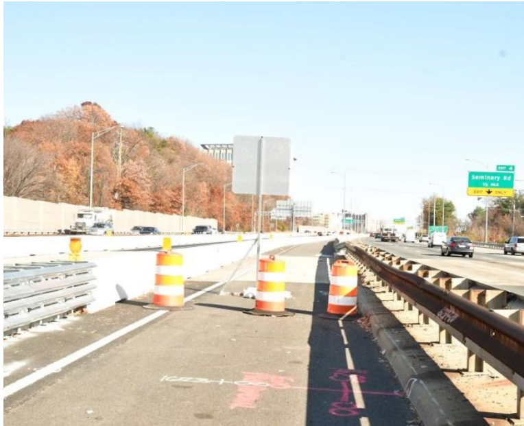
Establishment of a work zone in preparation for future construction along the I-395 HOV lanes.
