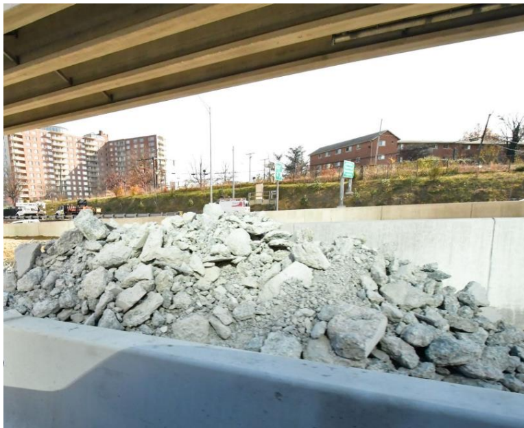
Spoils from the demolition of a concrete island along the southbound I-395 general purpose lanes near Seminary Road.
