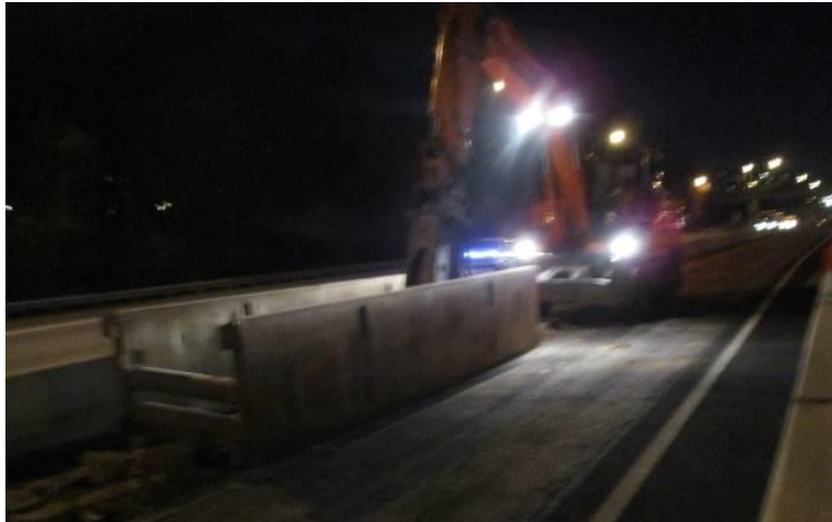
Concrete Island demolition in preparation for future construction work on the I-395 Express Lanes.
