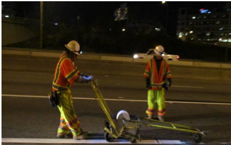
Pavement Marking Tape installation in preparation for a traffic shift along the northbound I-395 general purpose lanes.
